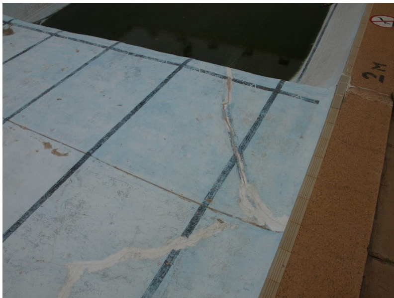
MAJOR CRACKING AND REPAIRS AT TRANSITION TO DEEP ZONE
