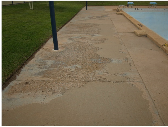
ERODED CONCRETE CONCOURSE
