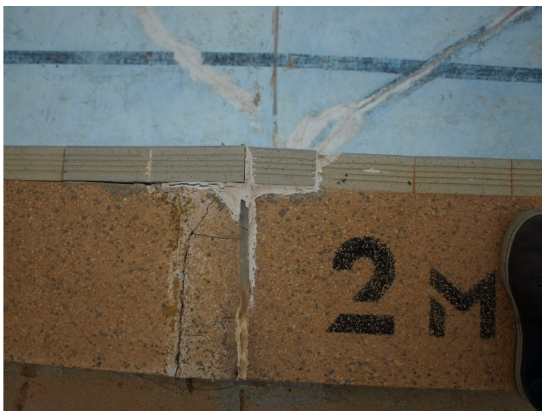
CRACKING AND HEAVING EVIDENT AT CONSTRUCTION JOINT
