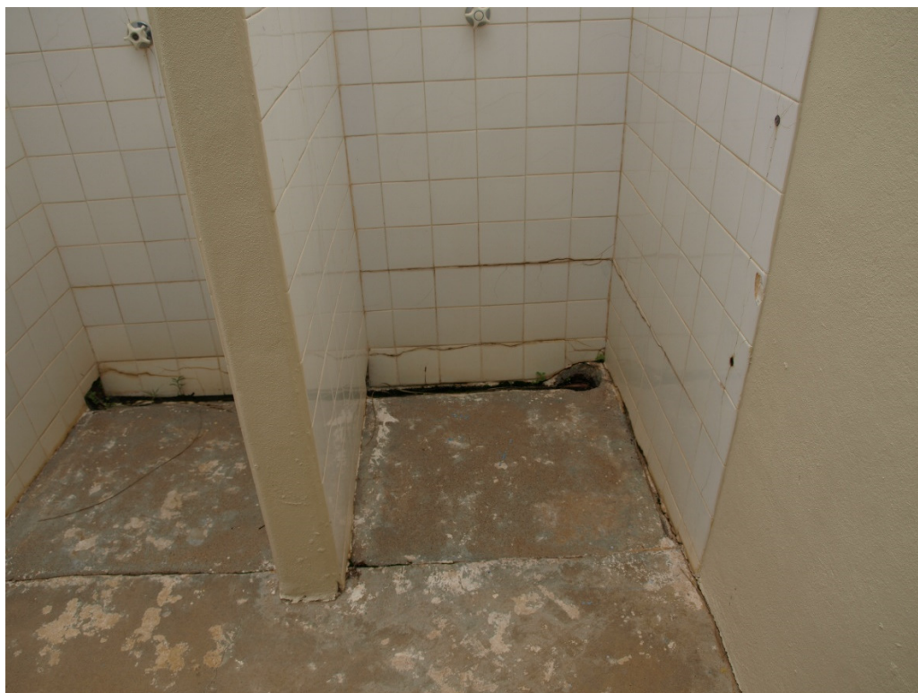
SHOWER CUBICLES - SUBSIDENCE, TILING AND FLOORING ISSUES
