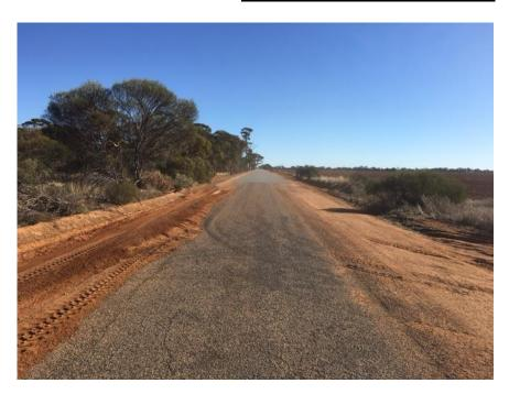
Widening and clearing of the S bends on Scotsman Road East of Bimbijy Road have been completed and we now have a 10m pavement width through the corners which should improve safety.
