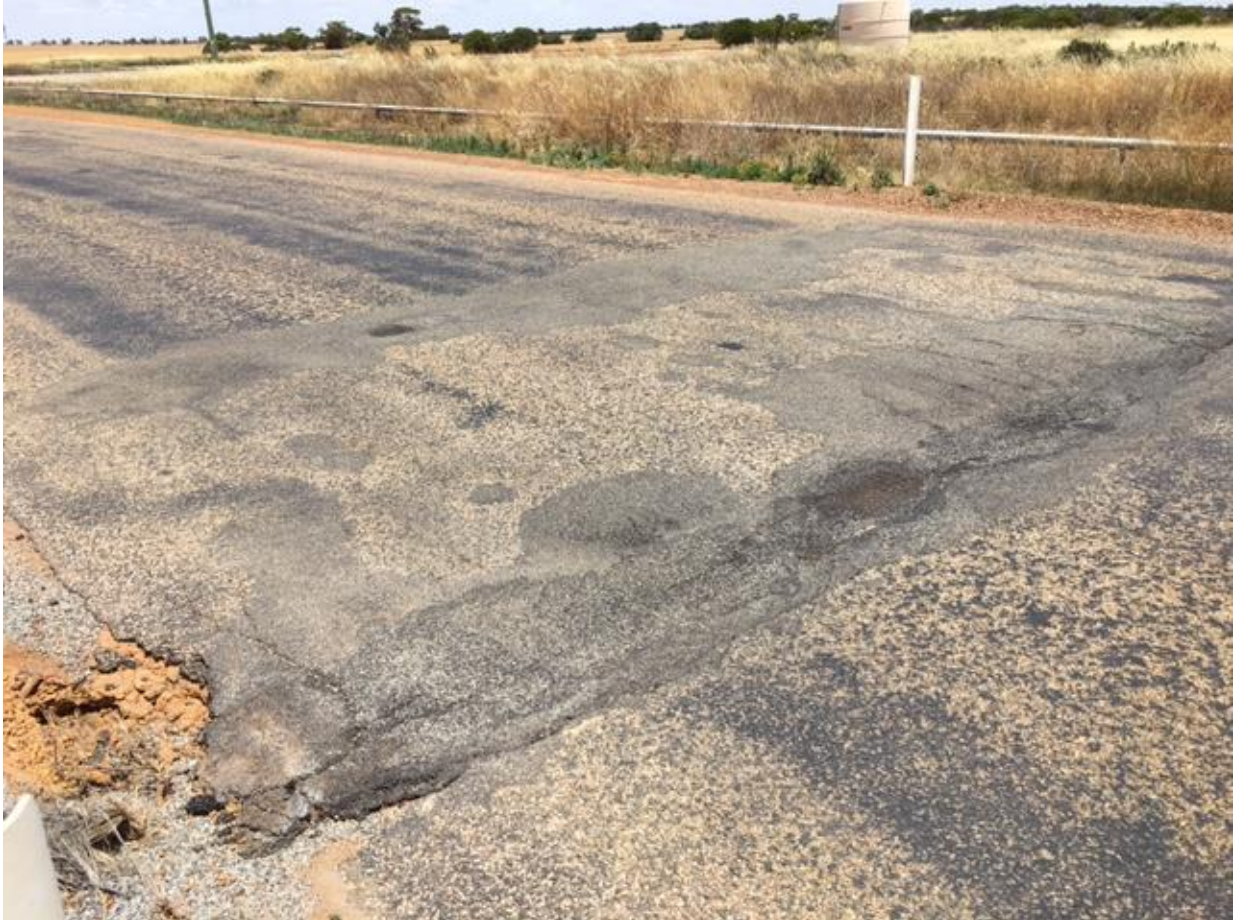
Above: Patched section at culvert, rough running surface, poor culvert condition.
