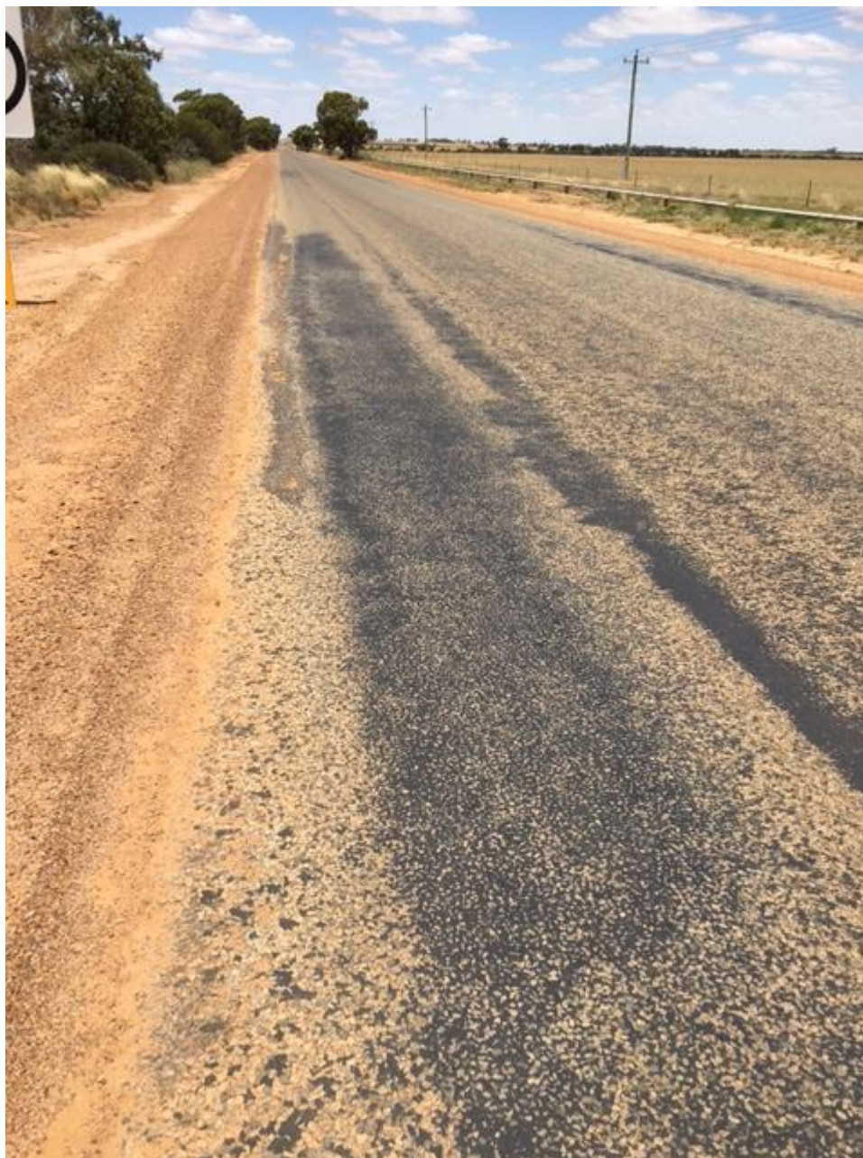
Above: Sunken section of road that pools water during rain events.
