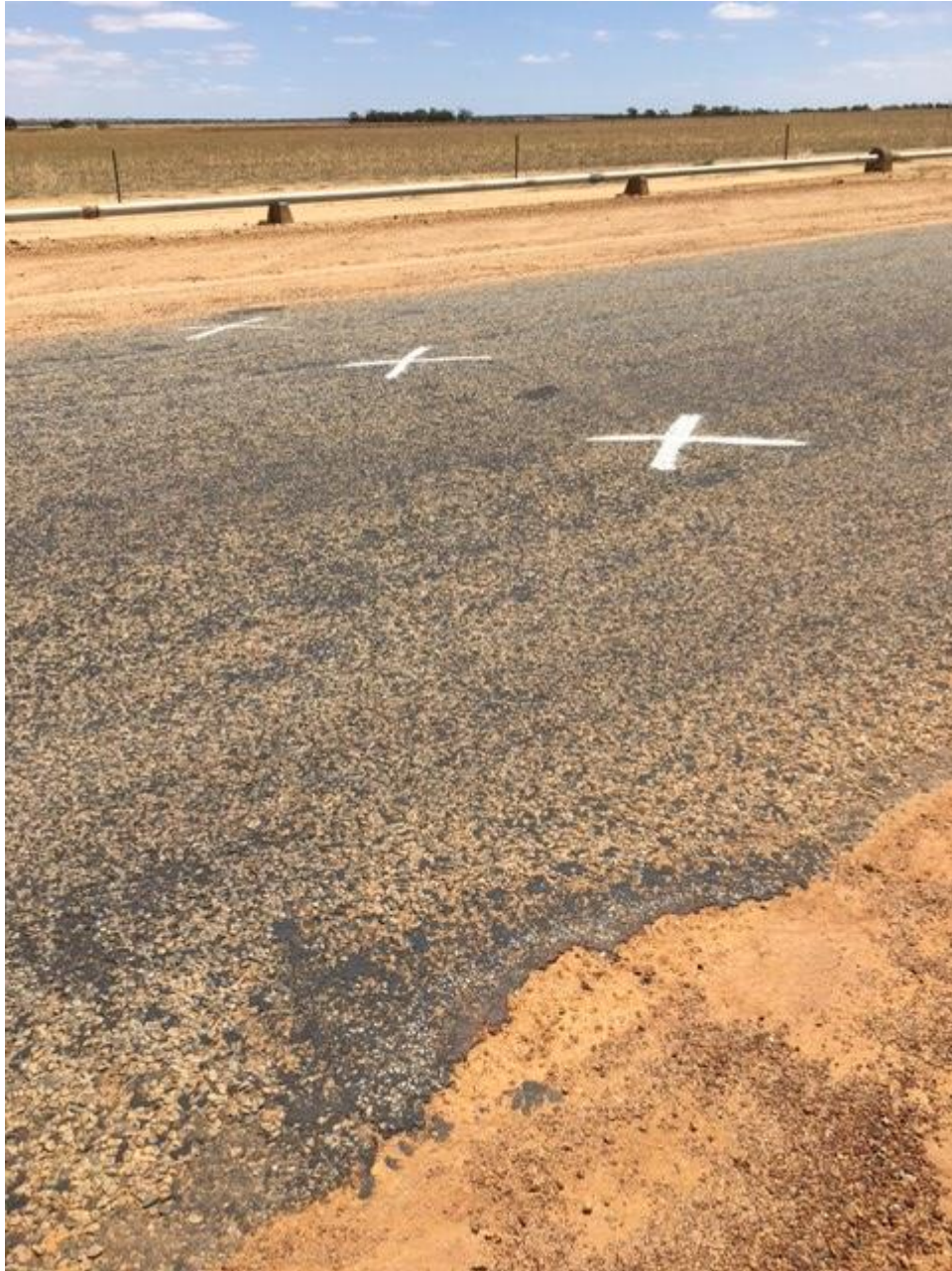
Above: Raised section of road and poor shoulder conditions
