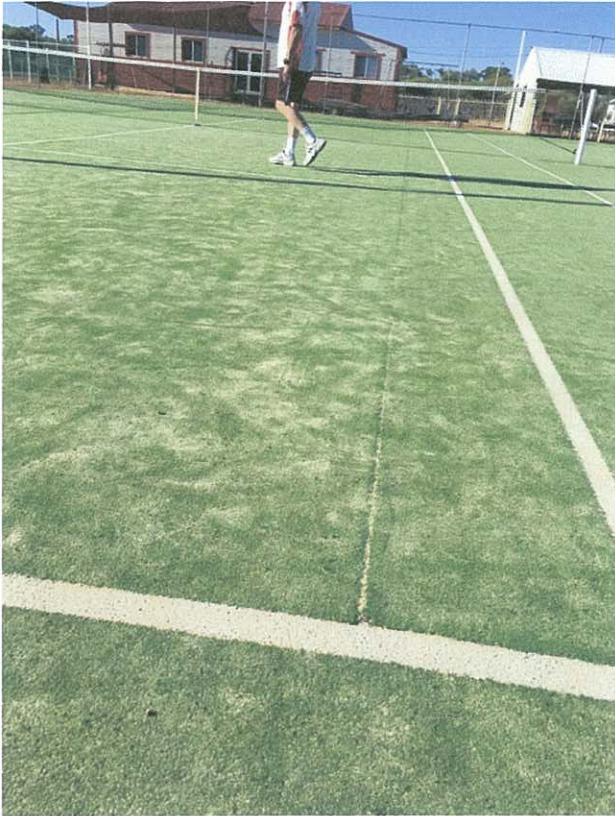
Joins between the rolls becoming visible on Court 1 (left photo) and Court 4 (right photo)
