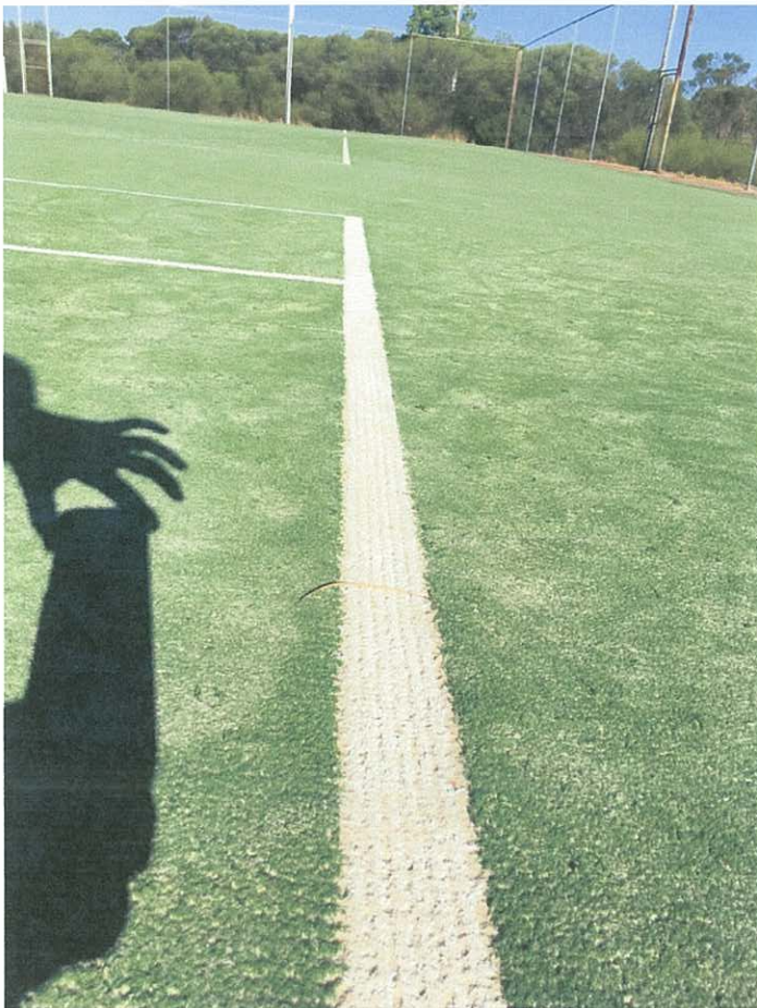
Joins between the rolls becoming visible on Court 1 (left photo) and Court 4 (right photo)
