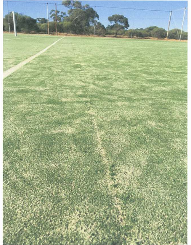
Joins between the rolls becoming visible on Court 1 (left photo) and Court 4 (right photo)
