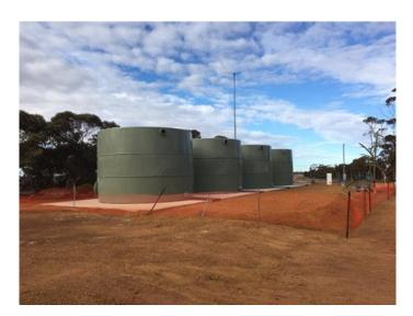
The new fence has been installed around the Beacon capture dam and the new tanks for Beacon Rock have been installed. Once the tanks are plumbed and brought into service which is expected in the next 2 weeks the Shire will take control of the old AA tank at Beacon Rock.
