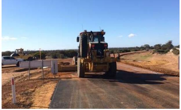
Beacon-Bencubbin Road intersection has been finalised to pavement standard and is now waiting for primer seal, kerbing and asphalt to complete works.
